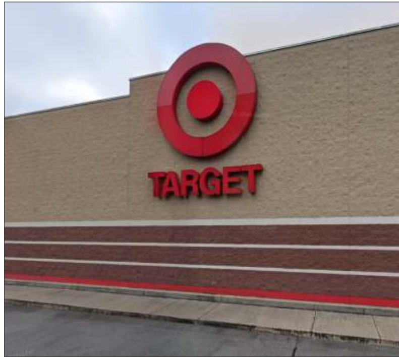
PHOTO SURVEY OF EXISTING CONDITION
